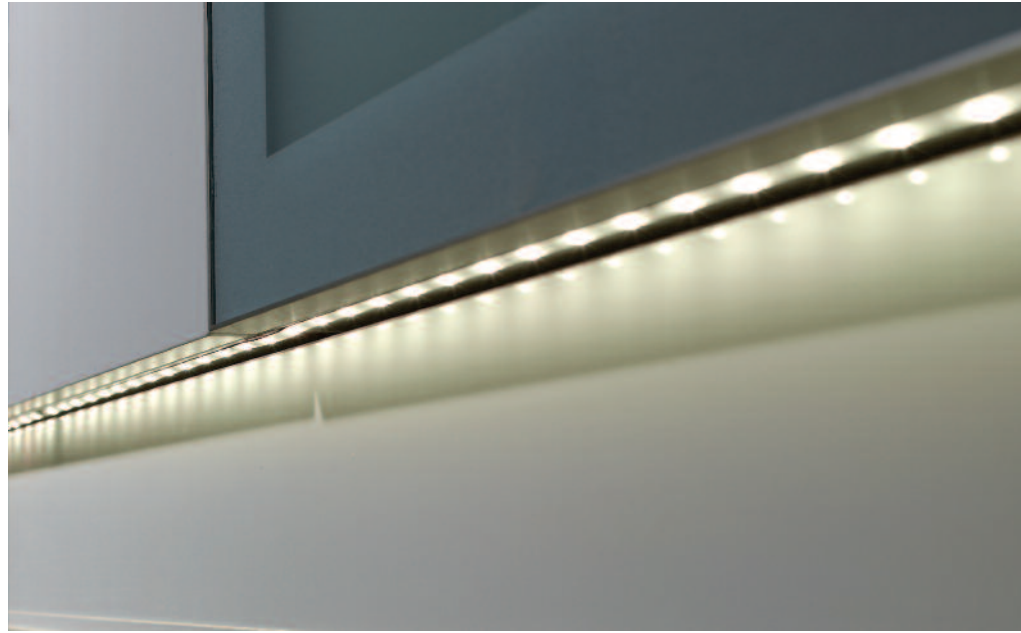
Flexible strip lighting
